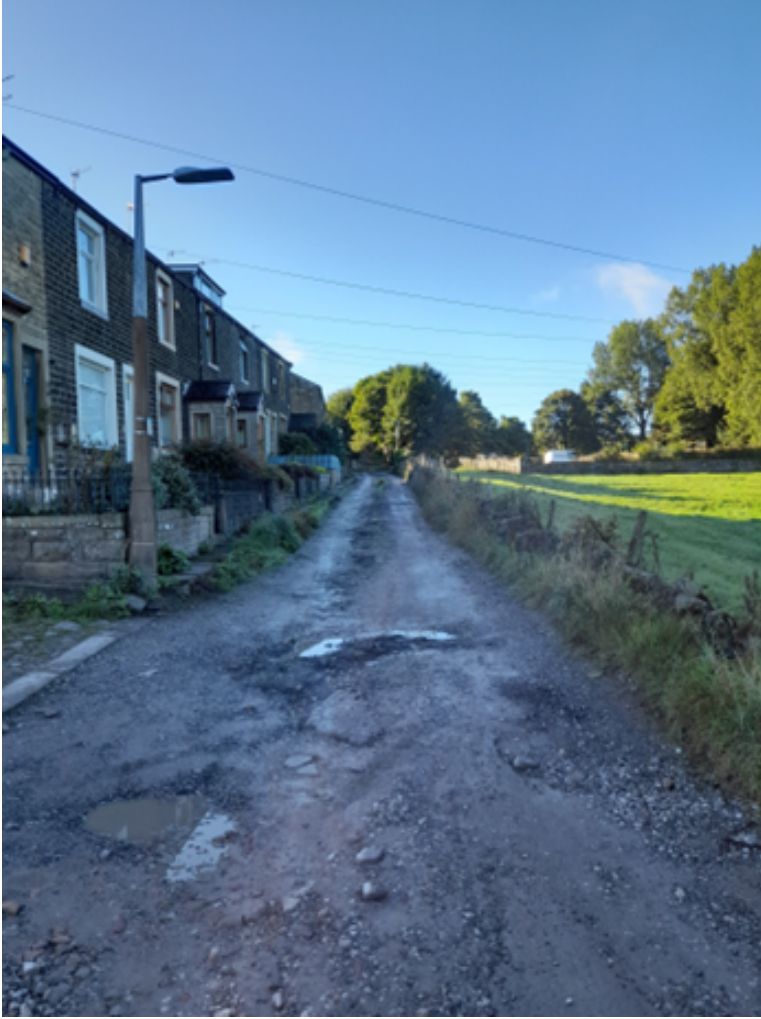
Fig 2a: Access Road viewed south from the site
